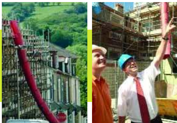
Construction work on homes in East Lancashire
