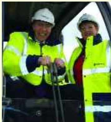
ODPM Minister Keith Hill, with NewHeartlands Chief Executive Pauline Davies, at the Bootle building site
