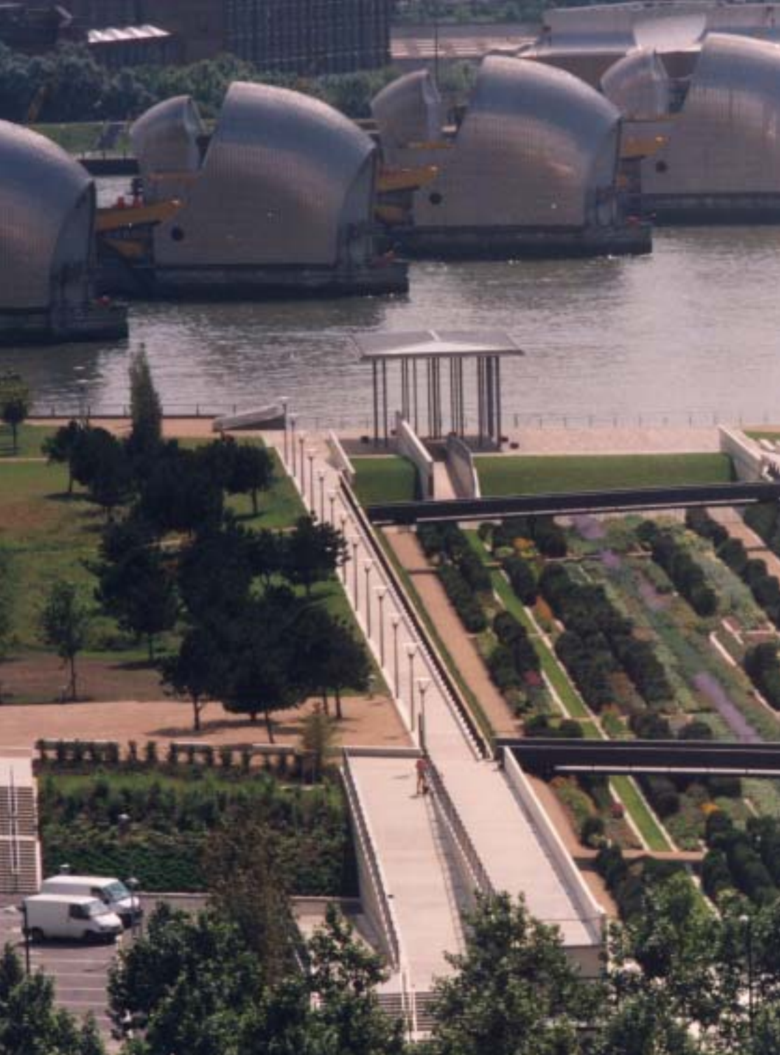
Thames Barrier Park
