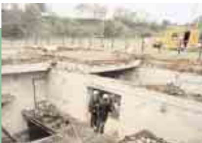
Abbeystead pumping station explosion
