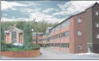
Mill House, Surrey Place, Guildford. A Constructing Excellence demonstration project.
