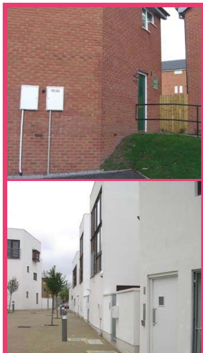
Figures 33 and 34: Two examples of how a lack of attention to the detailed arrangement of these 'interface elements' can have a very detrimental effect on the visual quality of places (Dominic Church).
