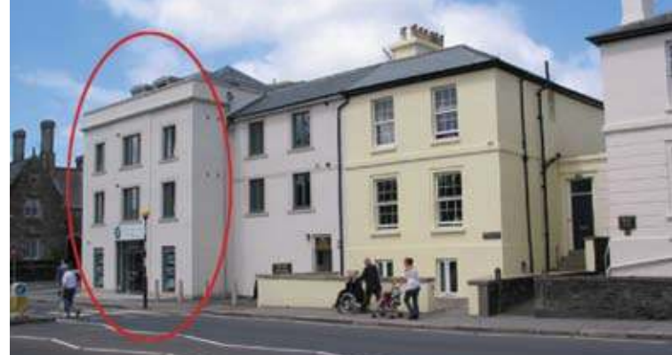
Fig 5: The new scheme (highlighted) was designed to be sympathetic to the adjoining Georgian buildings (HATC / Jan Randall).
