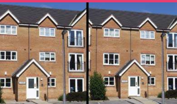
Figs 39: 76% of RSL development staff polled preferred the right elevation where the first floor windows are bigger (HATC).
