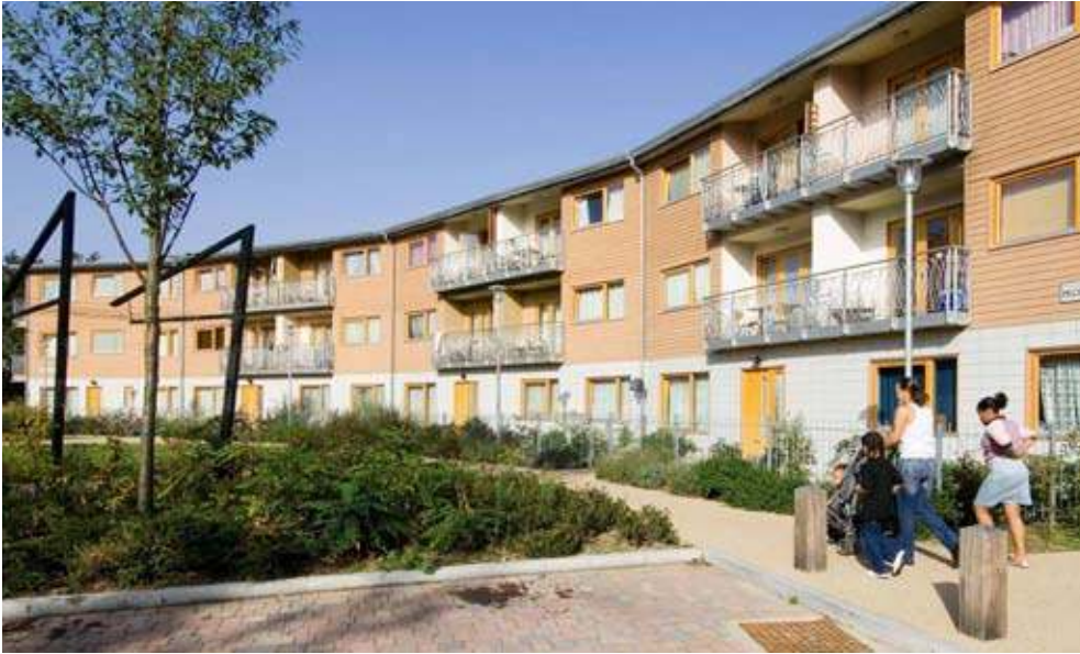
Eco homes in south London (Source: CABE/David Millington)
