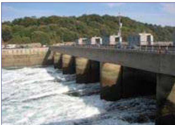
Figure 11 La Rance tidal barrage
