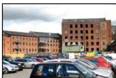
Left: The Congleton Silk Mills are being transformed as part of a major local development.
