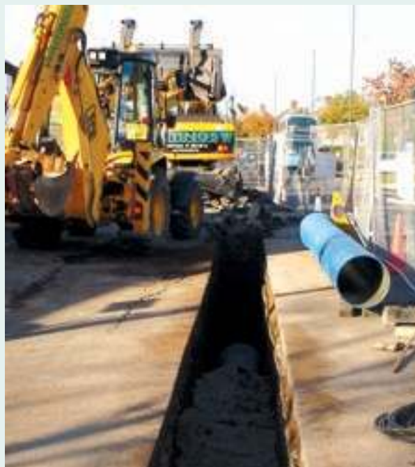
Figure 2.9 Aspley Lane street works
