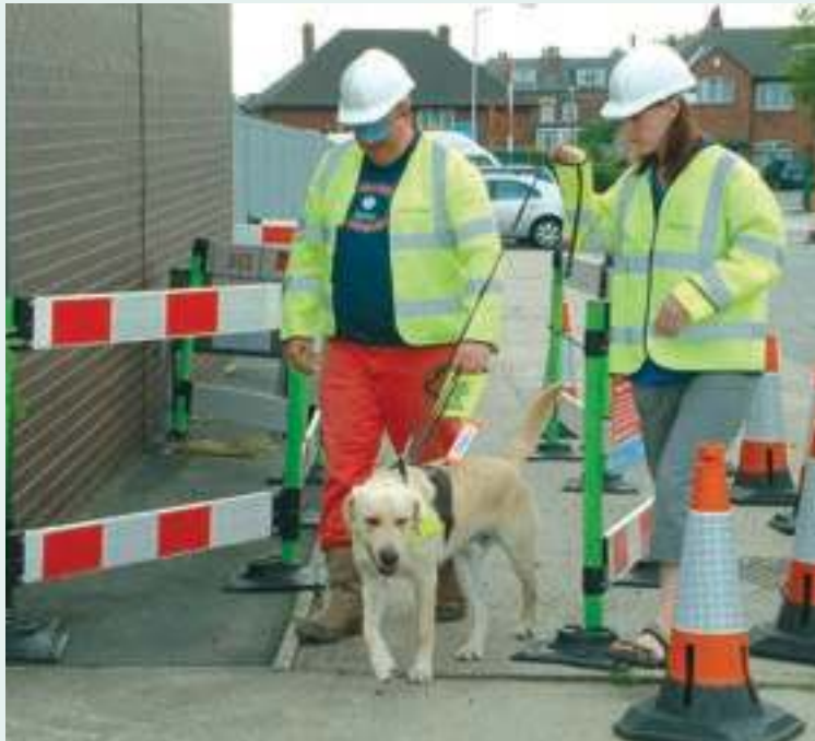
Figure 3.1 Guide dog and trainer walking a street works site
