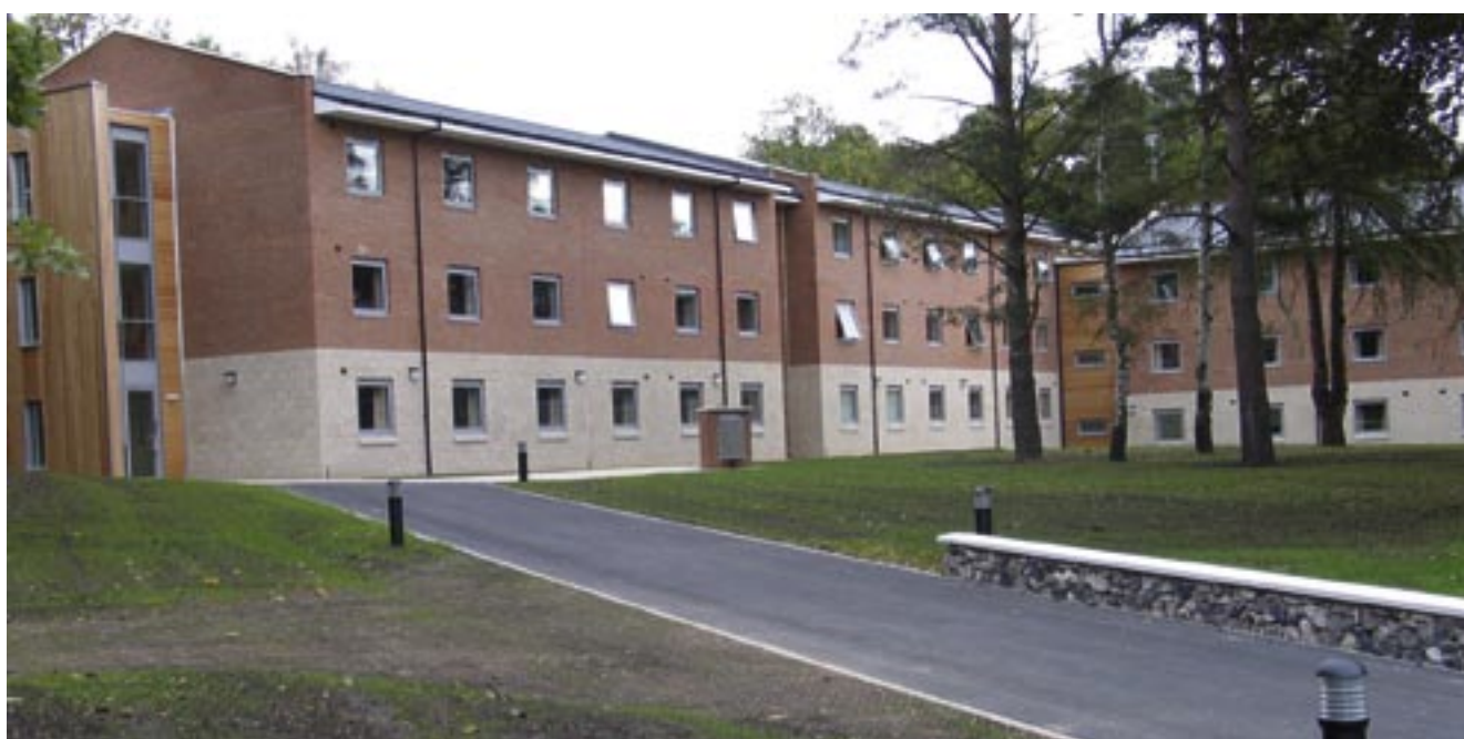
New accommodation built under the Single Living Accommodation Modernisation contract
