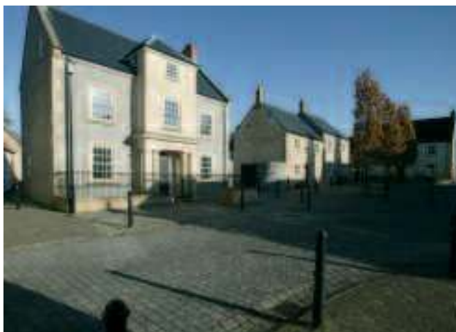
Far left Parking is provided through driveways and courtyards Left A pedestrian-friendly environment has been created Right Open space is overlooked from adjacent buildings
