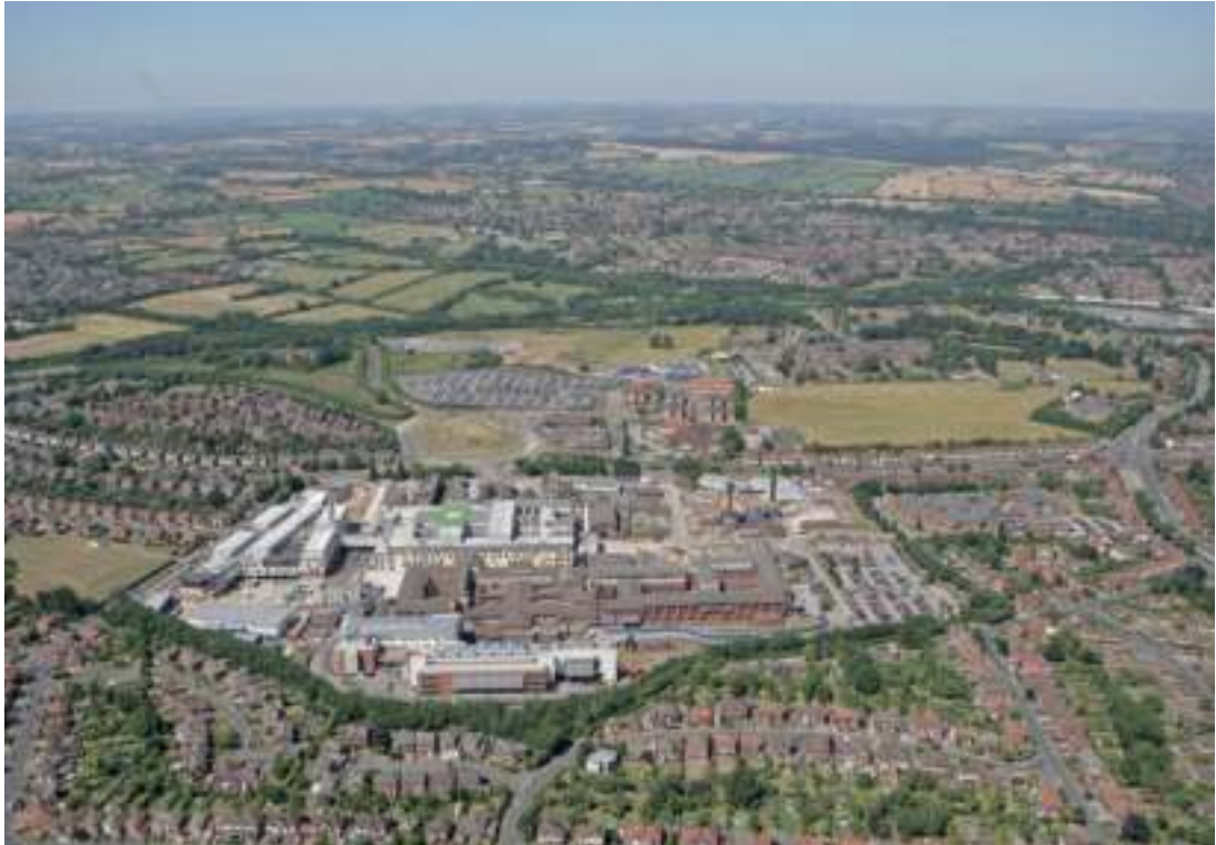
■ Aerial view of the Derby City General Hospital including Phase 1 of the new build - August 2006
