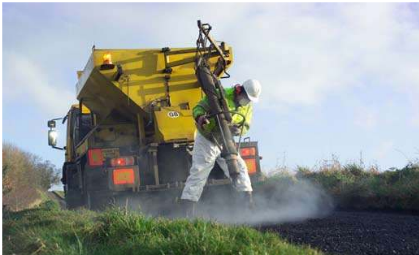
Maintenance work in Northamptonshire Source - Atkins
