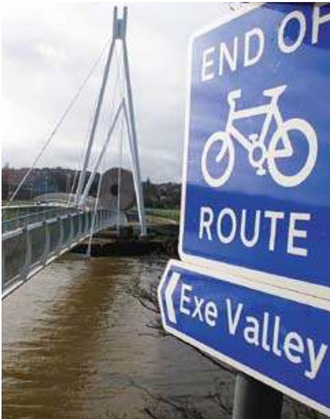
Millers Crossing over the River Exe at Blackaller Weir, close to the centre of Exeter Source - Devon County Council
