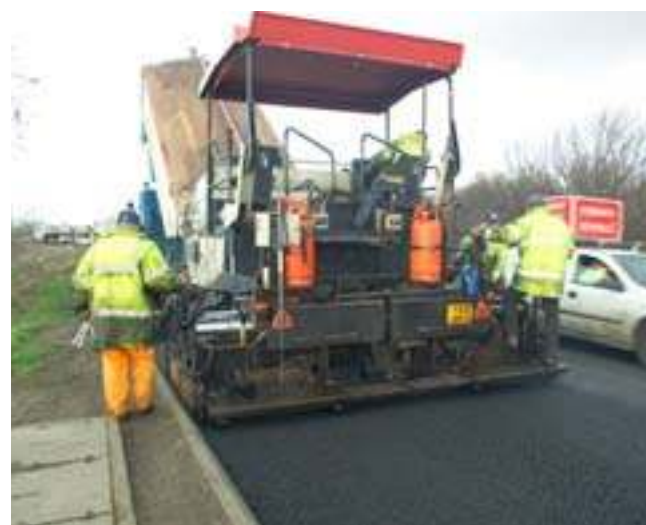
Maintenance work in Northamptonshire Source – Atkins
