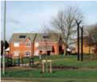
Low-rise, suburban housing in Castle Vale
