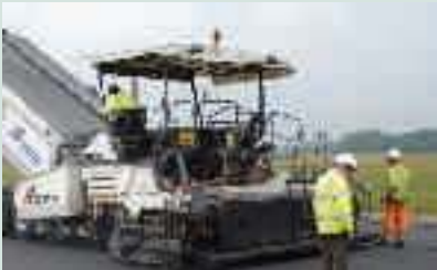
Final coat of Marshall Asphalt, RAF Linton-on-Ouse
