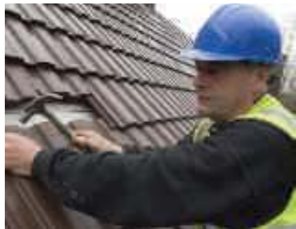
The 500 th new roof to be fitted under the 2007/08 SFA re-roofing programme
