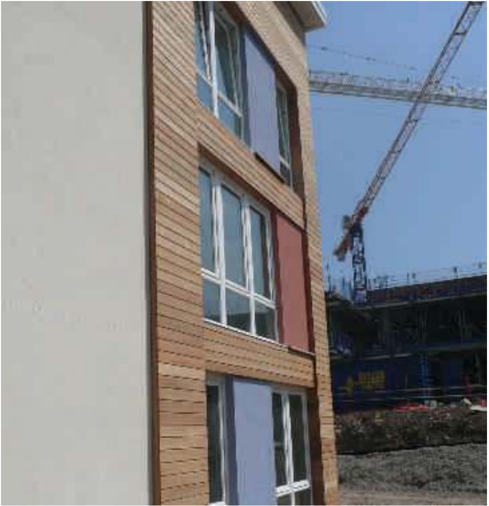
SLA and Headquarters under construction, PJHQ Northwood
