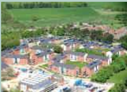
Solar panels, Junior Ranks SLA, Swinerton Barracks, Perham
